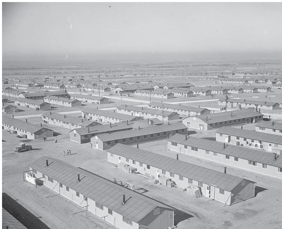
Overlooking the Amache Relocation Center near Granada, Colorado. In the foreground is a typical unit consisting of 12 six-room apartment barracks buildings, a recreation hall, laundry and bathhouse, and the mess hall. Photo by Parker, Tom. Amache, Colorado, 12/9/42.
